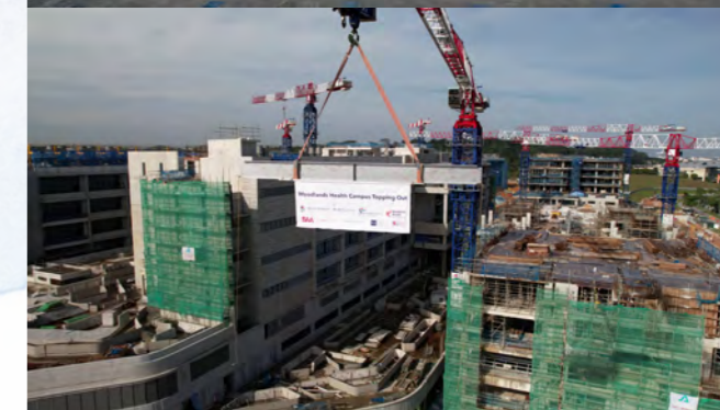
Woodlands Health Campus Topping Out event on 12 February 2022
